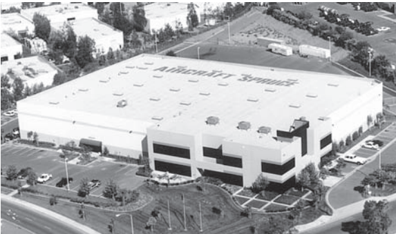
Present Home of Aircraft Spruce West (225 Airport Circle, Corona, CA.)
